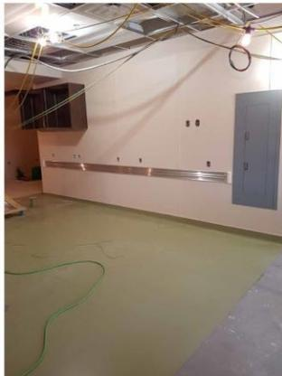
Shown: Central Nurse Station. Flooring in progress. Vinyl wall protection in place, millwork and guard rails in progress
