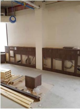
Millwork being installed at all patient treatment stations. The millwork serves as a chase for plumbing and electrical work.
