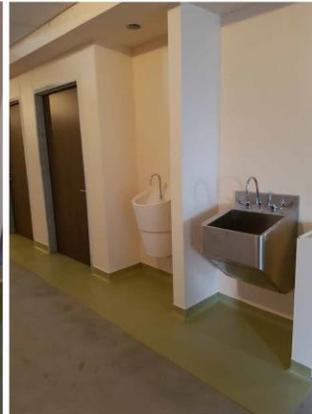
Inner core from treatment room. Utility sink and handwash in place. Flooring in progress
